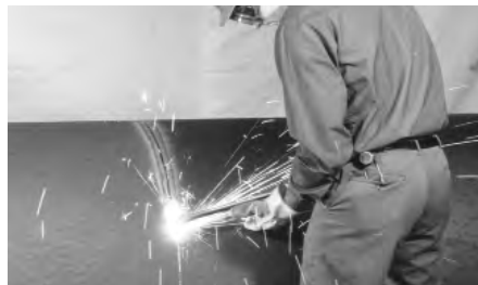
Cutting ductile iron pipe with torch.
