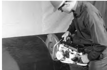
Cutting ductile iron pipe with abrasive wheel.
